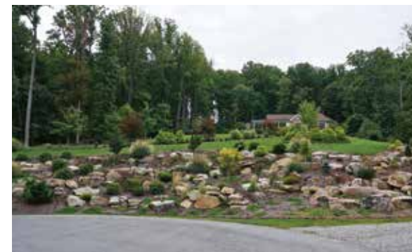
The mountainous Virginia landscape can create quite a challenge for Anderson and his crew. However, the company works to create solutions exemplified in this embankment, which has been stabilized by boulders and ornamental plants.
